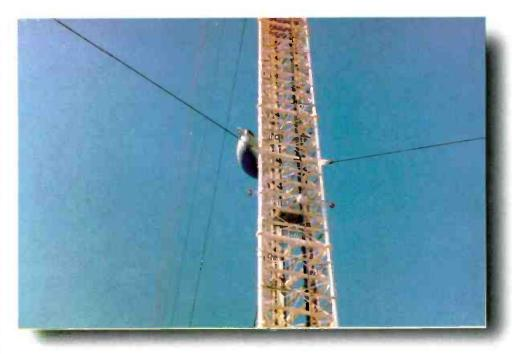
Intermediate tower lights can no longer be installed on the tower. Existing towers are "grandfathered," but new towers must have two fixtures installed so that at least one light is clearly visible without any obstruction from the tower members.
